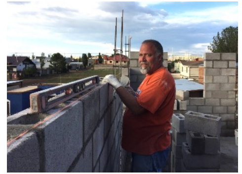
Dave Eldridge laid over 800 cement blocks!
